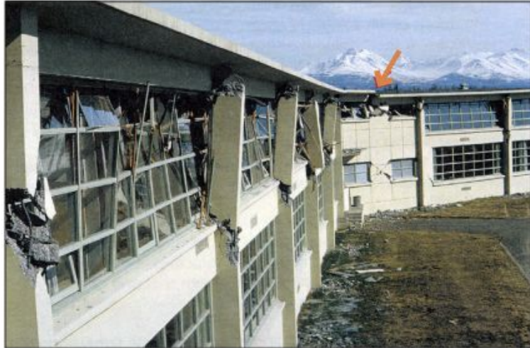
Concrete column failure, West High School, Anchorage, AK After 1964 Great Alaska Earthquake
