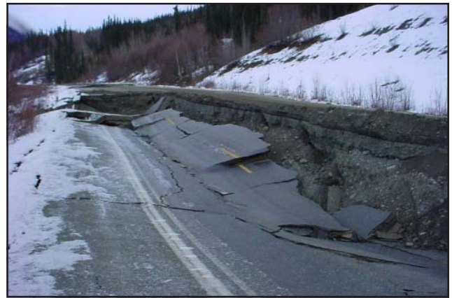
Figure 4. Highway damage along the Tok Cutoff during the magnitude 7.9 2002 Denali fault earthquake.
