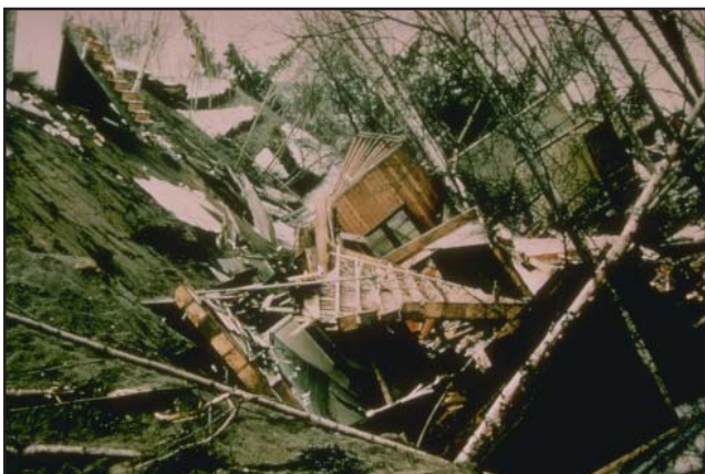
Figure 1. Destruction of homes in the Turnagain Heights subdivision of Anchorage during the 1964 earthquake.
