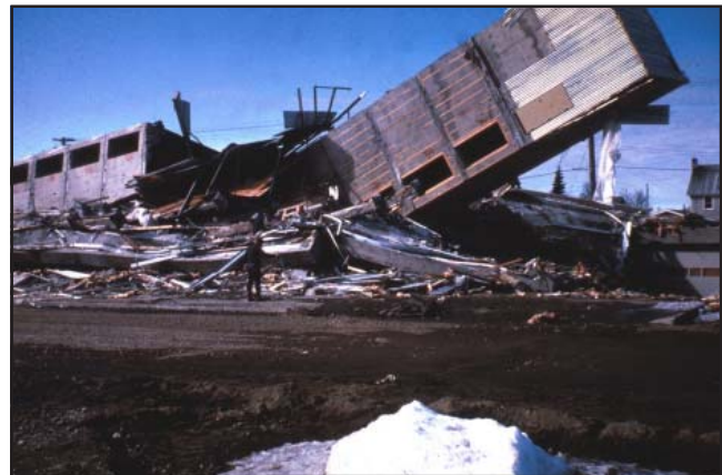
Figure 2. Collapse of the newly completed Four Seasons Apartment Building in Anchorage during the 1964 earthquake.
