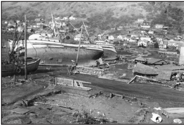
Figure 3. Tsunami damage in Kodiak resulting from the 1964 earthquake.
