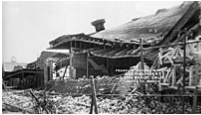
Figure 2. Damage to Franklin Junior High School in Long Beach, 1933
