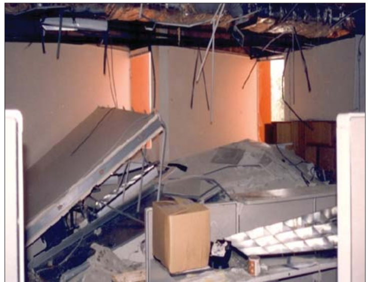
Nonstructural partition wall, ceiling and lighting damage, Northridge, CA, earthquake, 1994 (FEMA photo)
