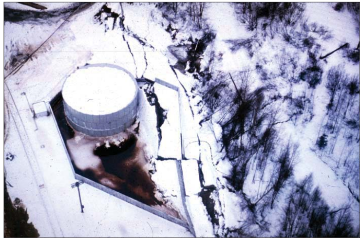
Ruptured fuel tank in Anchorage, 1964 Earthquake (USGS photo).
