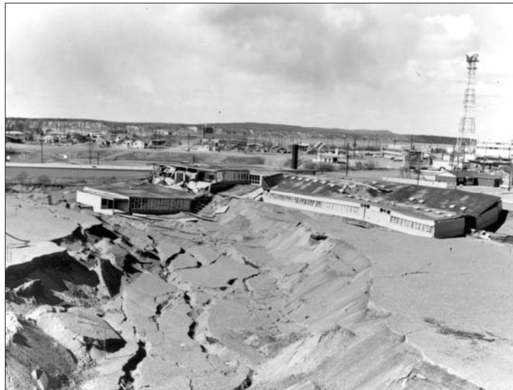
Government Hill School, 1964 earthquake (USGS photo).
