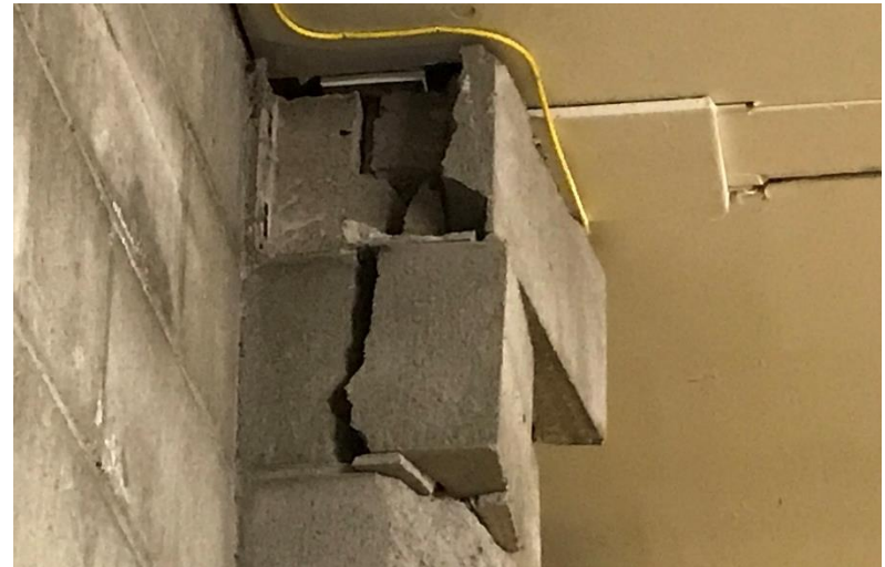
CMU damage at Wasilla Police Station (Above) and at Whitney Road Warehouse (Below)
