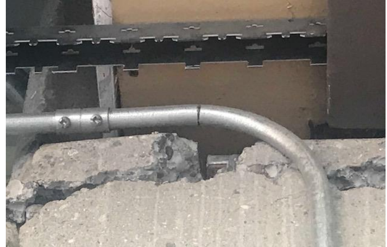
CMU damage at Wasilla Police Station (Above) and at Whitney Road Warehouse (Below)
