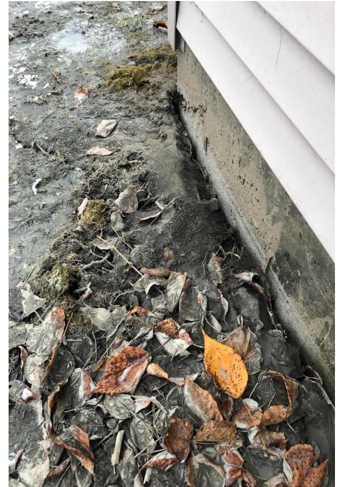
DOT&PF Annex Building
