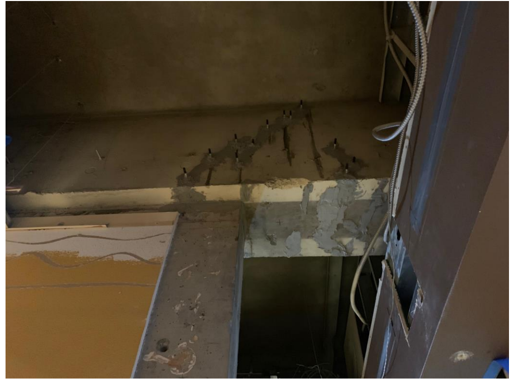
Concrete girder shear cracking Aftershocks effect
