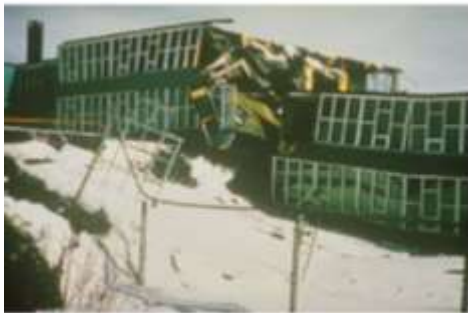
Government Hill Elementary School after the 1964 Earthquake
