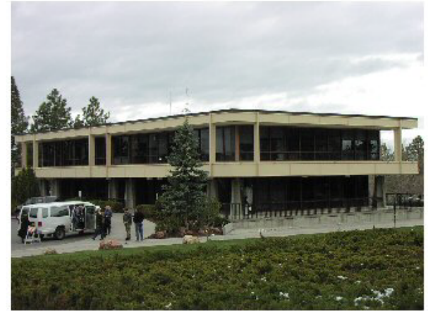
Admin. Bldg. at Oregon Institute of Technology where numerous buildings were damaged in 1993 quake
