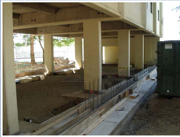
WOU HSS building: Soft-story collapse hazard
